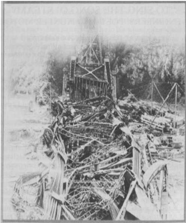
THE COLLAPSED QUEBEC BRIDGE, 1907
